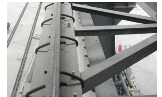
Bu lông móc kẹp ray Anchor bolts for rail clamp
